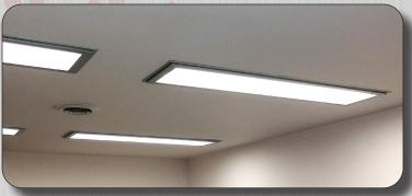
Paramount's **Techniseal® Grid Series** is designed to seal to the T-Bar ceiling material. Our standard troffer is built for a 1" (15/16") Standard T-Bar and requires **no grid suffix** be added to the part number. If the grid system requires the G0, G1, or G2 option, please supply the grid manufacturer & model number when ordering.
